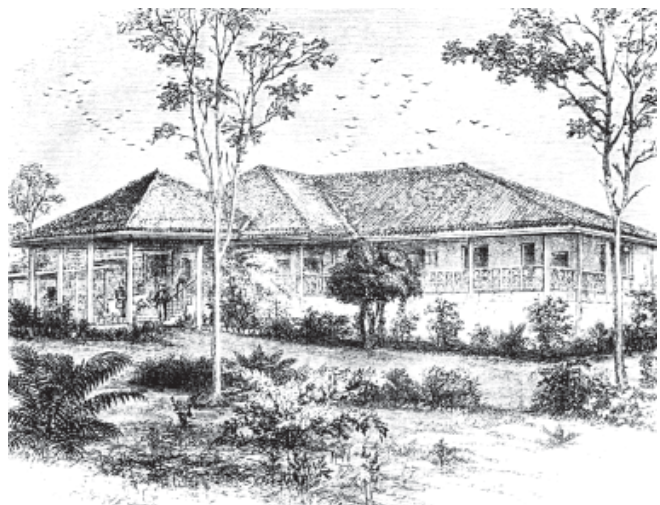
Fig. 12.23 A bungalow in Bombay, nineteenth century
